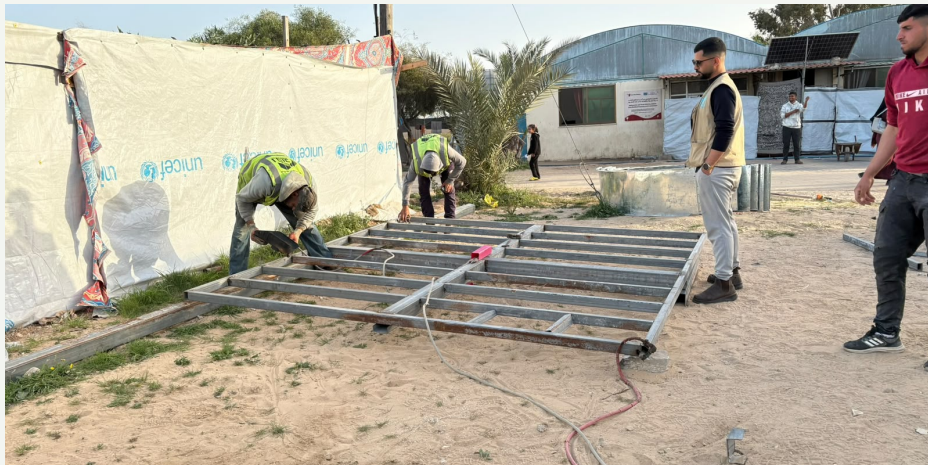
STRUCTURAL WORKS AND SITE PREPARATION
